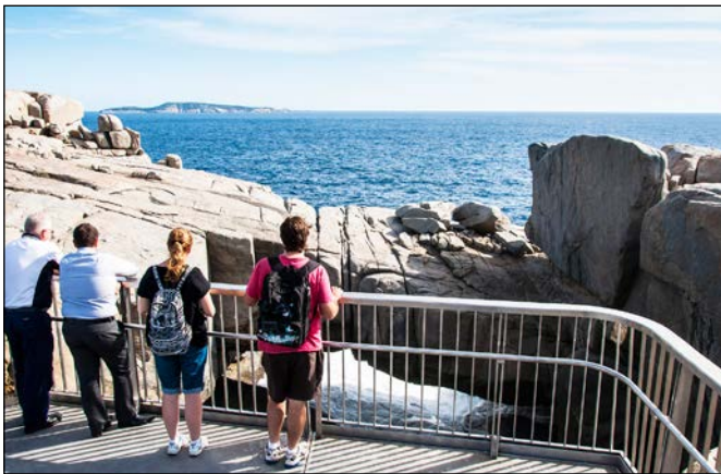
Upgraded infrastructure at the Natural Bridge.
