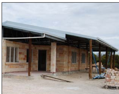
Restoration work at the Twertup Field Studies Centre is almost finished.
