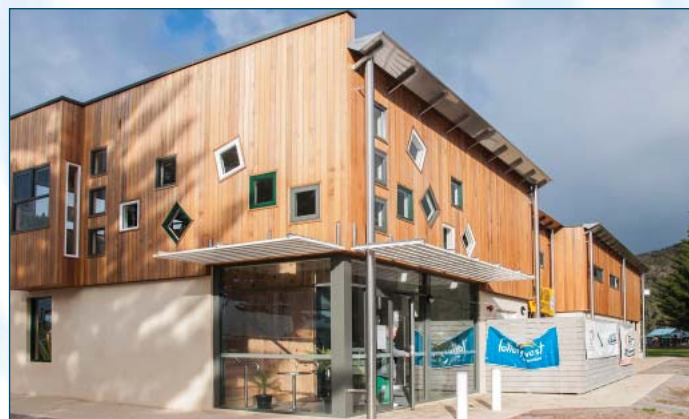
Albany Surf Life Saving Club's improved premises at Middleton Beach.
