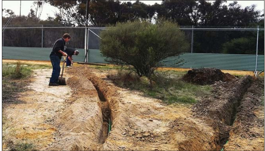
Yongergnow volunteers Barry Savage and Tim O'Neill dig cable trenches for the fowlcams installation inside the malleefowl aviary. Photograph by Vicky Bilney.
