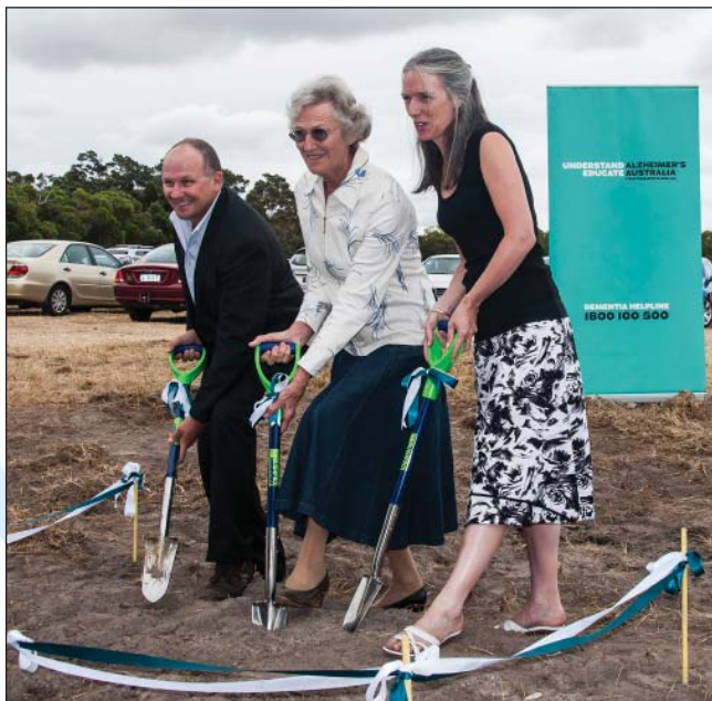
South West MLC Colin Holt, Hawthorn House community member Jo Dart and Hawthorn House program manager Elizabeth Barnes turned the soil to start construction of the new premises.
