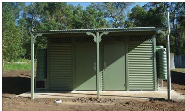
New facilities at Torbay Hall will cater for walkers, horse riders and Munda Biddi Trail cyclists.
