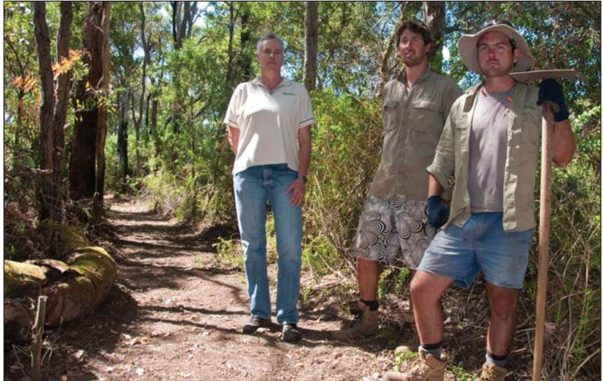
Munda Biddi Trail coordinator Kerstin Stender with construction supervisor Brett Trouchet and assistant supervisor Peter Horsington on a section of trail near the Sleeman River.
