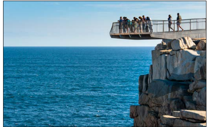
Upgraded infrastructure at The Gap in Torndirrup National Park.
