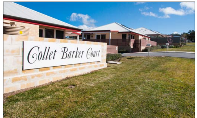
The Collet Barker Court project is providing accommodation and facilities for independent seniors in Mount Barker.
